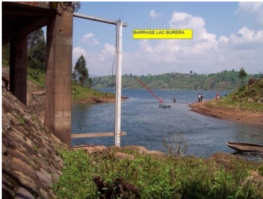
Figure 31: Water level decline in Lake Burera which supplies Hydropower plants of Ntaruka and Mukungwa
