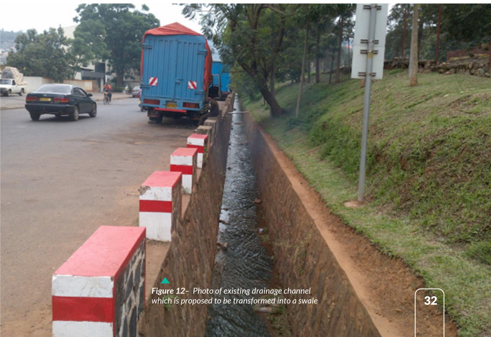
Figure 12- Photo of existing drainage channel which is proposed to be transformed into a swale
