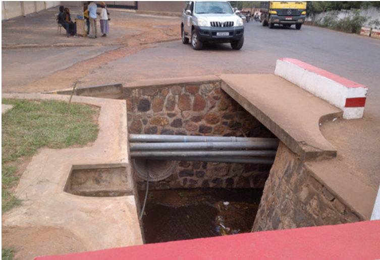
Figure 32 RM-07 existing culvert
