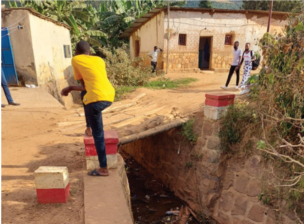
Figure 30 RM-02 existing wooden bridge
