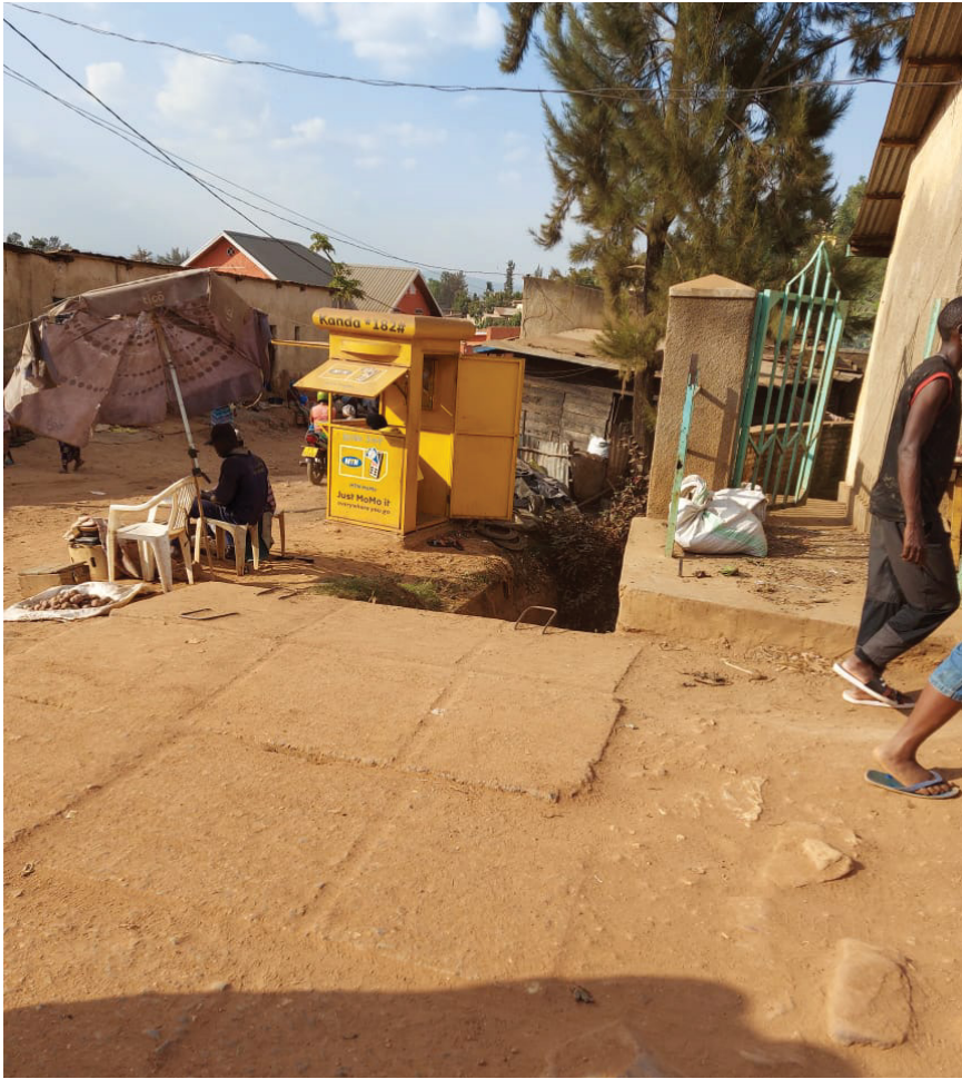
Figure 28 RM-01 existing culvert
