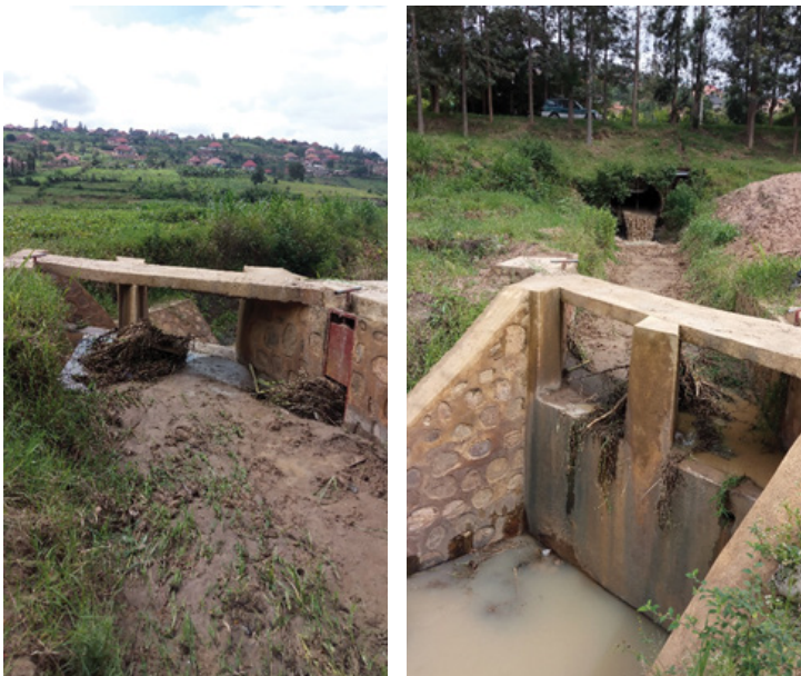
Figure 26: BI-001 current state at the existing intake structure
