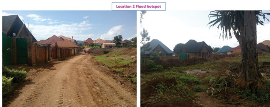
Figure 3: Location 2 flood hotspot in Gihundwe
