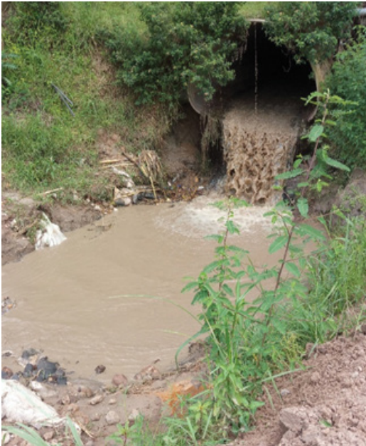
Figure 25: BI-01 current state at the exit of the existing pipe culvert
