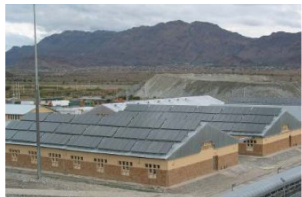
Figure 6.3: Solar water heating installation at Anglo Platinum's Brakfontein change-houses [24]
